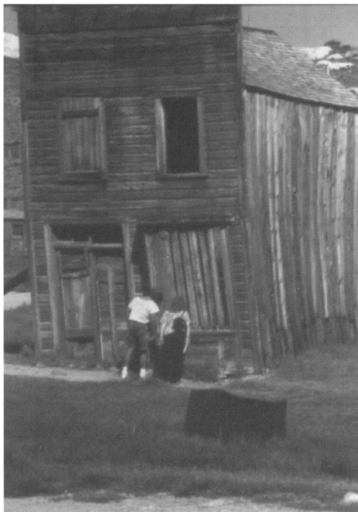
Figure 6. Bodie State Historic Park is preserved according to a policy known as "arrested decay," where buildings are stabilized but not restored. Their apparent frailty and tarnished appearance persuade visitors and staff of the Park's authenticity. Though this building, the Swazey Hotel, appears to be falling down, it actually got a new roof (shingled in the style of the old one) in the mid-1990s.
